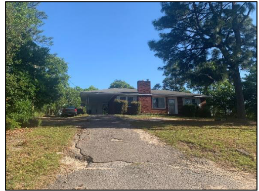
Single family home to the south on Dyches Road
